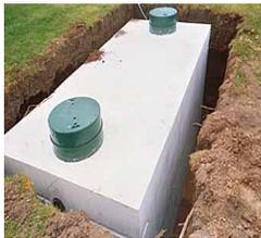
Newer cisterns are usually made from fiberglass or polyethylene, also with a riser for access from ground surface.
