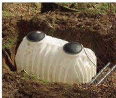
The access riser lid may look similar to that of a septic tank for the wastewater system. If you are not sure which riser lid is for the cistern, it may be helpful to find the septic permit site plan at Environmental Health Services.
